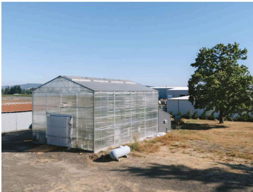
A Canopii greenhouse has a footprint of 2,500 square feet and measures 30 feet tall. (Canopii Photo)
