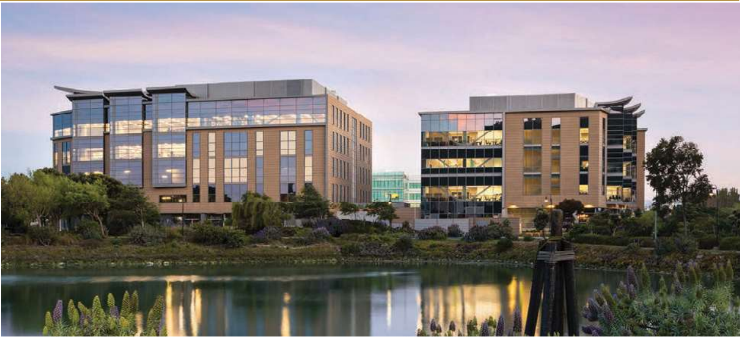
The Cove at Oyster Point, South San Francisco, CA LAB
